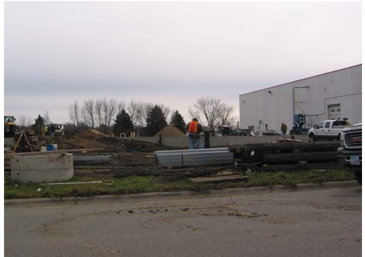
IFP, Inc., addition
