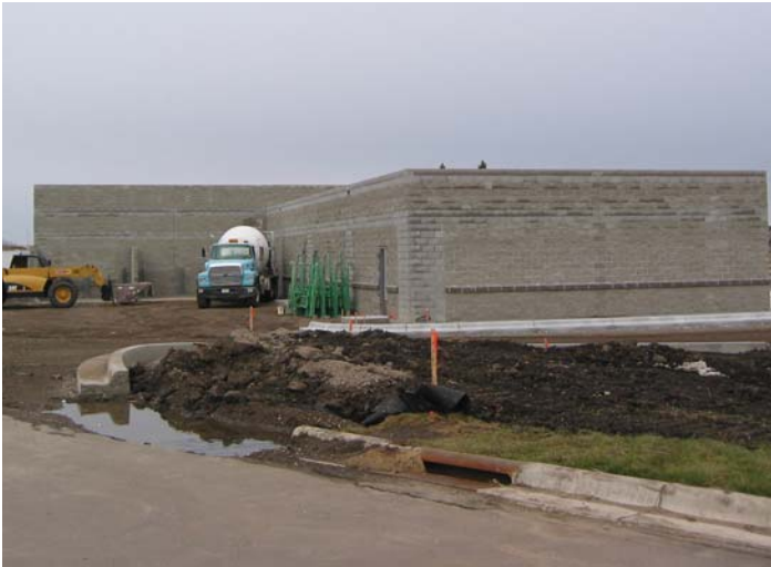
The Village Development (Haskell's), located at the intersection of TH 21 and 30th Street NW
