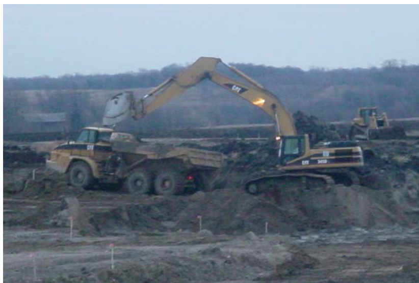
Aldi Inc. construction site
