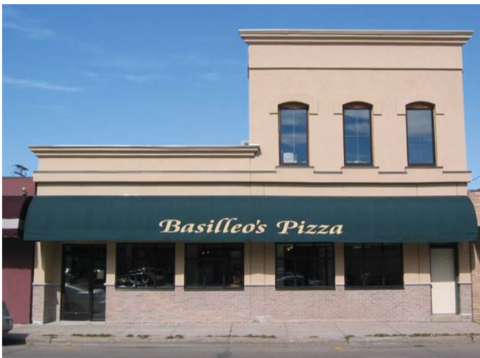
Basilleo's Pizza renovation
